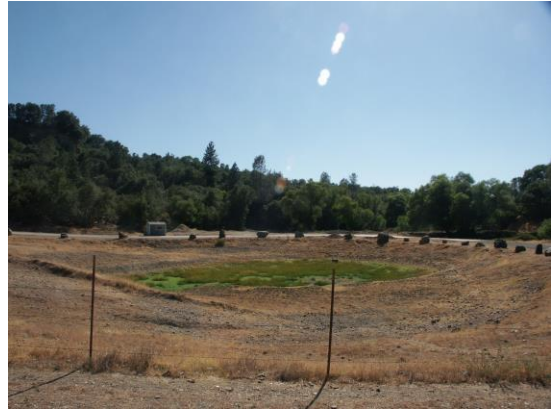
Photo 16 – lower detention pond
