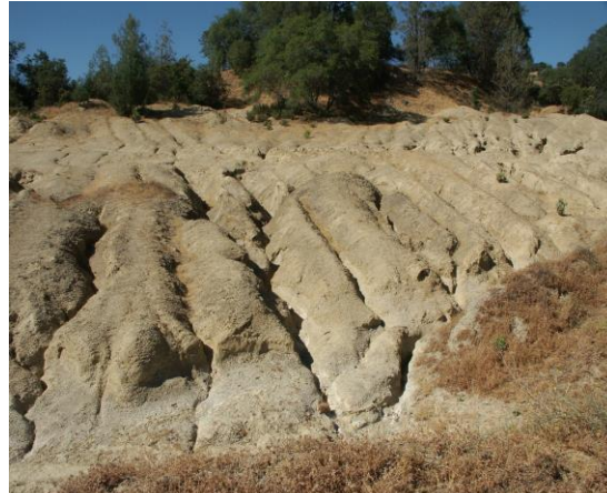
Photo 12 – eroding sand stockpiles
