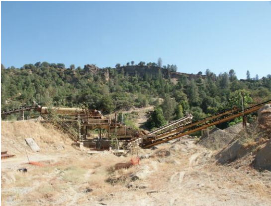
Photo 9 – gravel processing equipment
