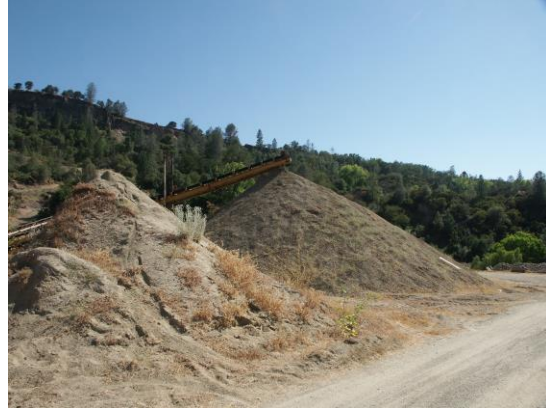
Photo 8 – gravel stockpile & equipment
