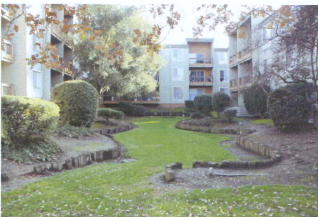
Photo 5 - Failing timbers at dog walk.
