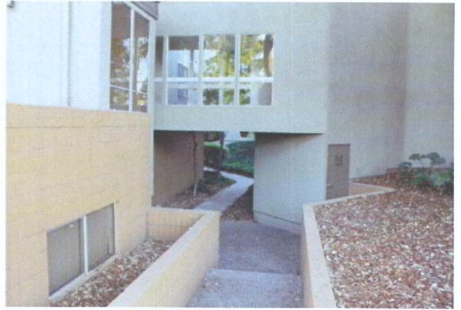
Photo 8 - Narrow, uninviting entry stairs.
