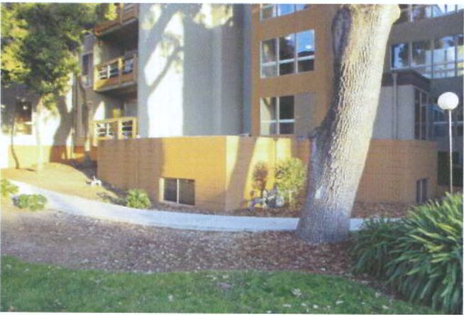
Photo 9 - Unattractive utility building at rental office walkway.
