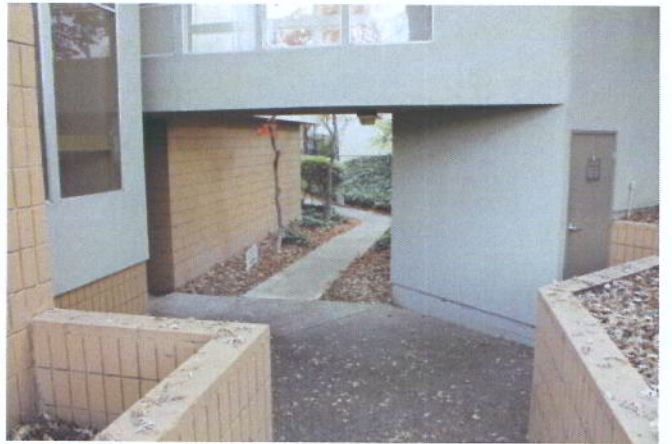
Photo 10 - Cameo view/walkway to pool area with light fixture.
